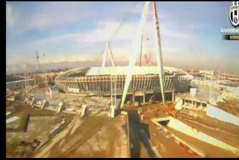
Teams should capture their stadium construction builds: http://bit.ly/pVKuL0
